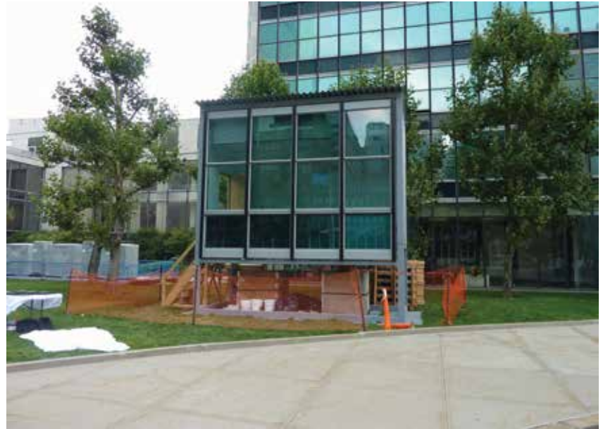
Figure 5. The curtain wall mock-up in front of the Secretariat Building, 2009 (Source: United Nations)
