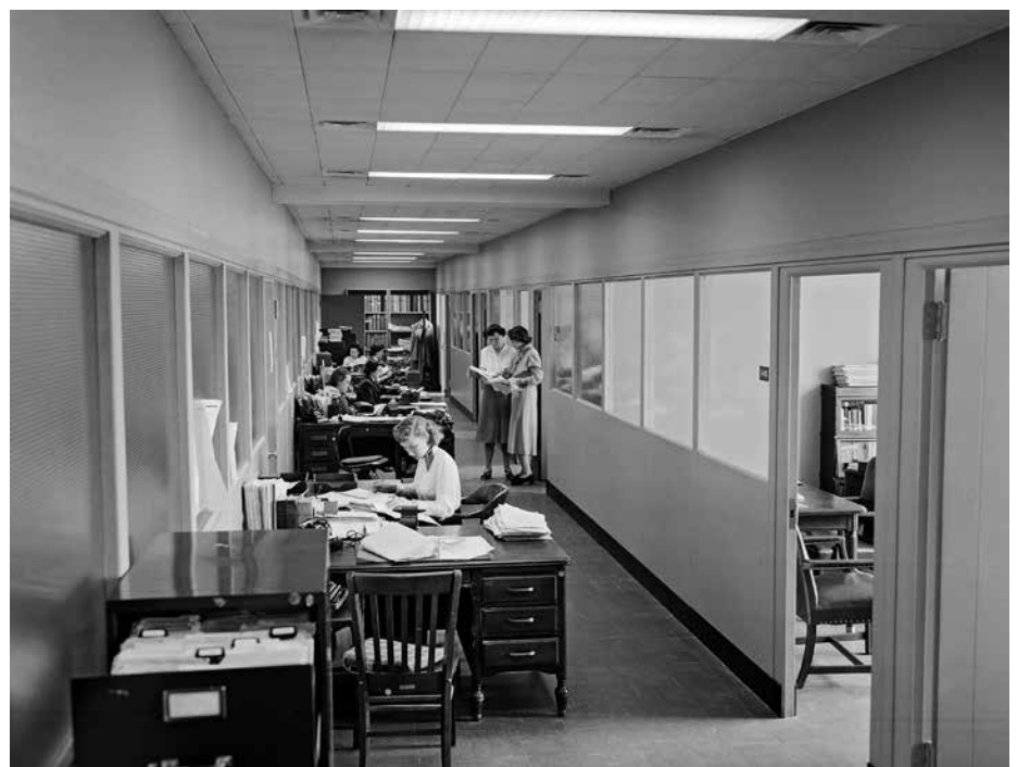
Figure 7. Floor-to-ceiling walls and doors for enclosed offices dominated the original layout of the floors in the Secretariat Building, 1951 (Source: United Nations)
