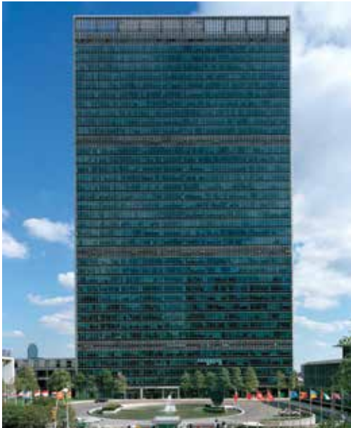
Figure 4. The curtain wall before the renovation - a patchwork in greenish hue, 2001 (Source: United Nations)
