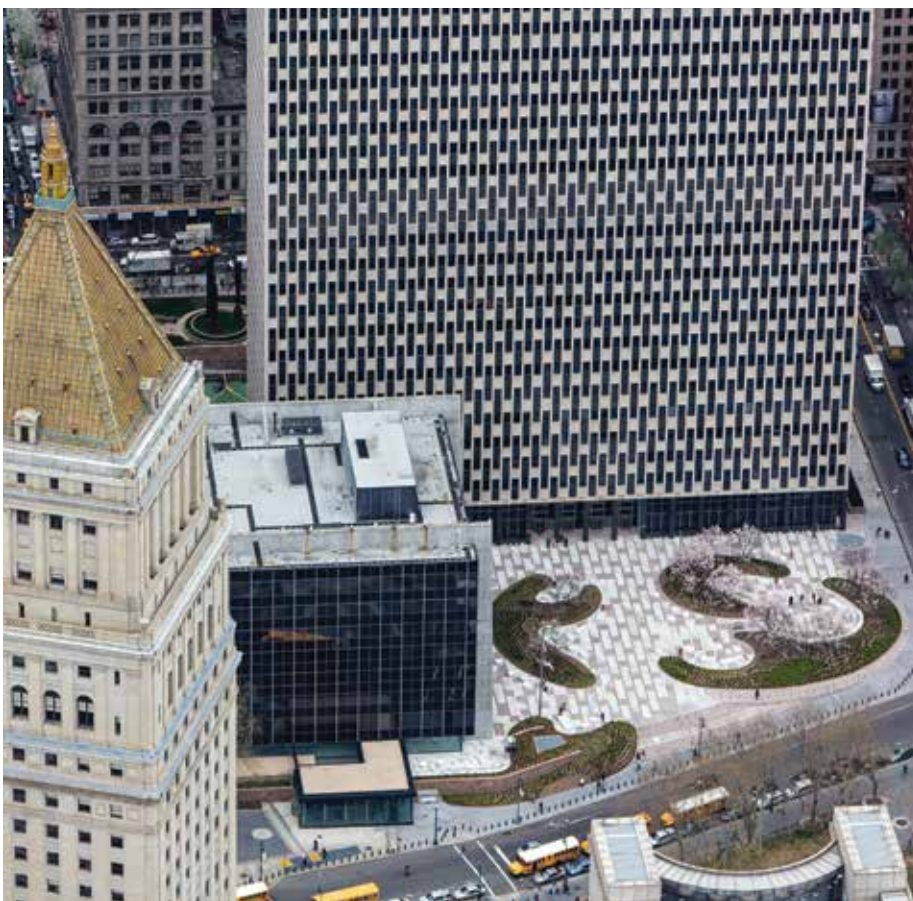
Figure 8. WASA/Studio A and Michael Van Valkenburgh Associates recreated the plaza topping the rooftop garage of the Jacob K. Javits Federal Building in New York (Source: Alex Maclean)
