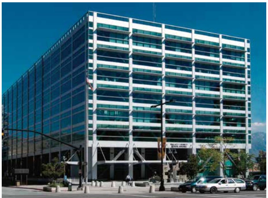
Figure 6. Wallace F. Bennett Federal Building in Salt Lake City, after the mid-century building underwent a seismic retrofit project that also replaced its curtain wall (Source: www.jabphoto.com)
