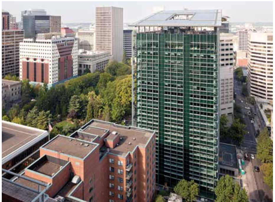
Figure 5. The modernization of EGWW culminates in a monumentally sized rooftop canopy integrated with 13,000 square feet of photovoltaics. The angled device is optimized solar exposure, and channels stormwater for collection (Source: Jeremy Bittermann)
