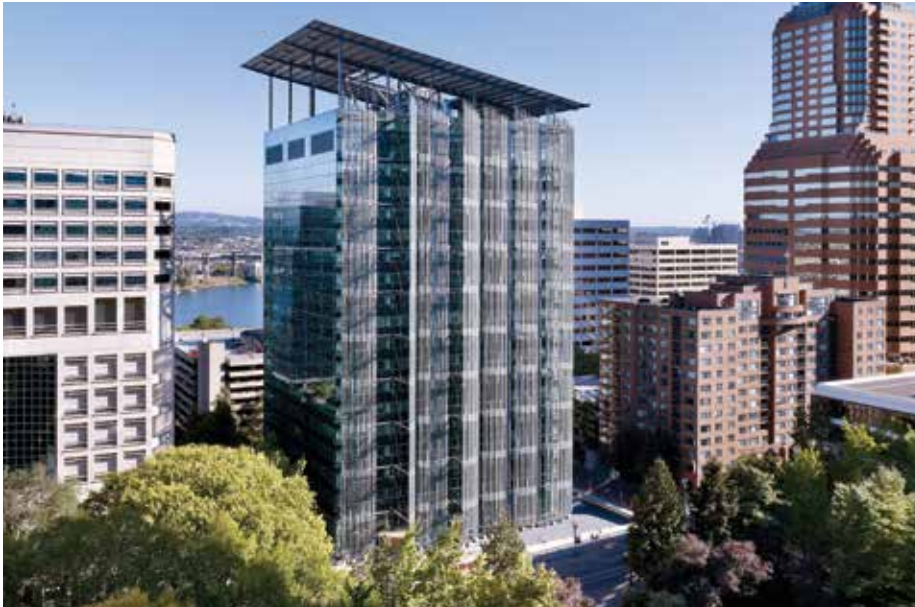
Figure 2. The north corner of EGWW reveals that the building's shading devices are precisely customized to orientation: the northwest elevation is shielded by 18-story tall aluminum reeds, while a more standard curtain wall faces northeast. (Source: Jeremy Bittermann)
