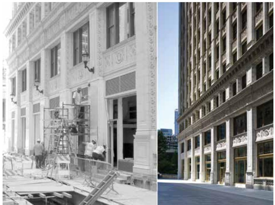
Figure 5. (Left) View of Wrigley Building facade before renovation; (Right) View of Wrigley Building facade after renovation. (Source: Goettsch Partners)
