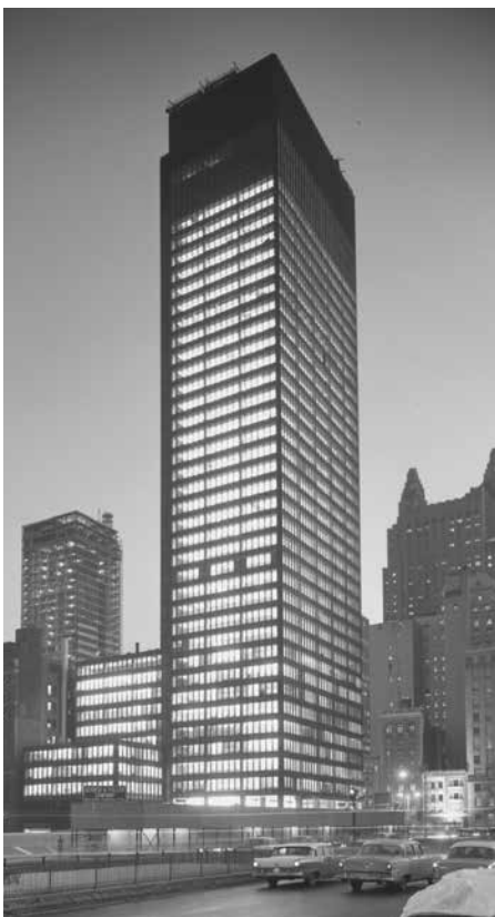
Figure 4. The Seagram Building, while an icon of modern skyscraper design, has three times the energy use intensity (EUI) per square foot than the Chrysler Building, according to 2013 Local Law 84 Benchmarking Data. (Source: Gottscho-Schleisner, I., 1958. Library of Congress Prints & Photographs Online Catalog. [Online] Available at: http://www.loc.gov/pictures/item/gsc1994027875/PP/ [Accessed 15 05 2015])
