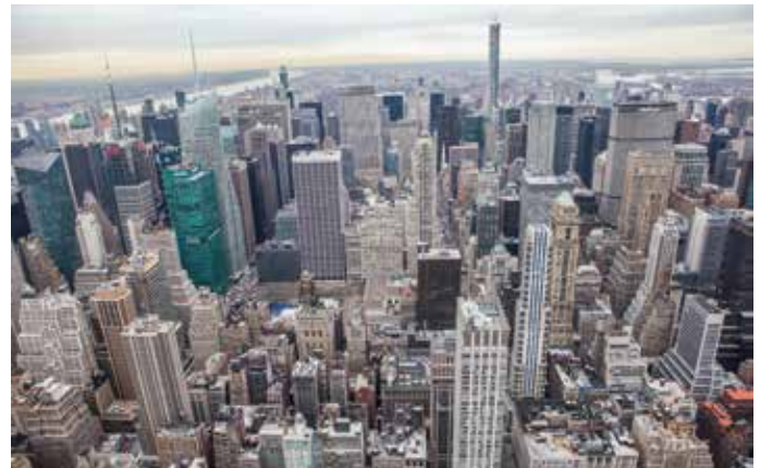
Figure 5. A view of Midtown looking north toward 432 Park Avenue. Many of these structures have potential for efficiency upgrades and repositioning. (Source: Quintano, A., 2015. Flickr.com. [Online] Available at: https://www.flickr.com/photos/quintanomedia/16335452951 [Accessed 15 05 2015])
