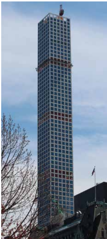
Figure 10. 432 Park Avenue includes 12-story clusters of apartments, separated by mechanical floors that act as gaps to reduce the wind pressure on the building. (Source: Suzuki, S., 2015. Flickr.com. [Online] Available at: https://farm6.staticflickr.com/5446/16572156763_6537afeecb_o_d.jpg [Accessed 15 05 2015])
