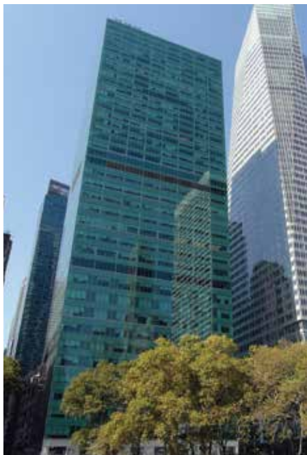
Figure 7. 1095 Avenue of the Americas is a 1970's office building that renovated its office space to Class A and re-clad its façade. (Source: Bastin, T., 2012. Flickr.com. [Online] Available at: https://farm9.staticflickr.com/8481/8191401072_83a54a4323_o_d.jpg [Accessed 15 05 2015])
