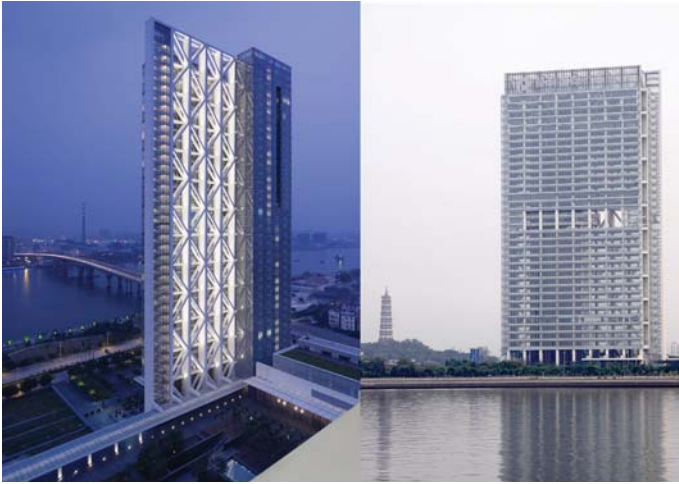
Figure 6. Perspective Views of Poly Real Estate Headquarters, Guangzhou (Source: SOM / Tim Griffith; SOM / Fu Xing)
