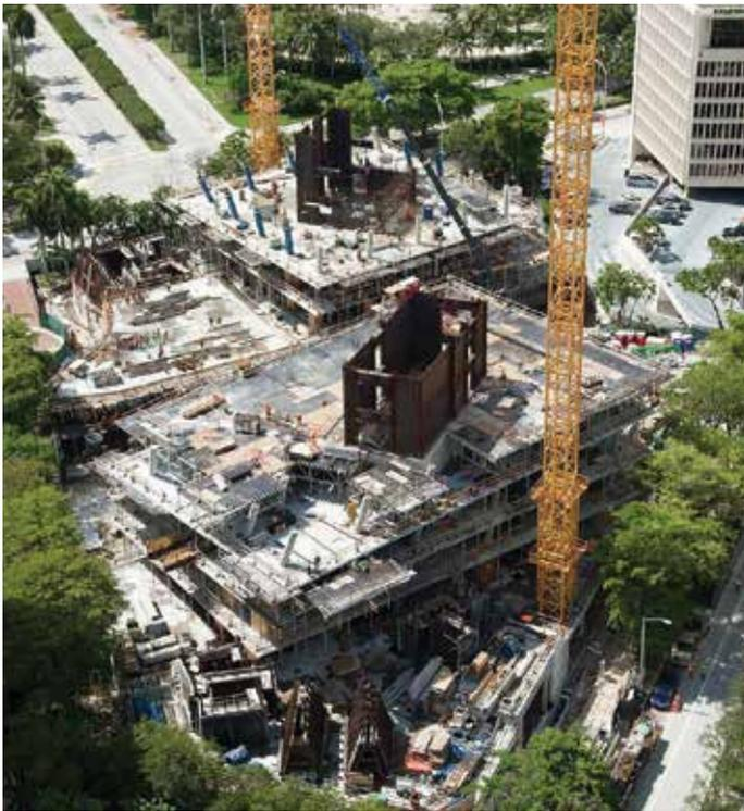
Figure 4. Aerial view of composite shear wall cores (Source: DeSimone Consulting Engineers, PLLC)
