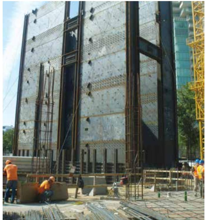
Figure 5. View of the steel plates within composite core (Source: DeSimone Consulting Engineers, PLLC)
