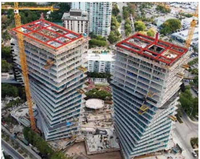
Figure 7. Roof girders highlighted (Source: DeSimone Consulting Engineers, PLLC)
