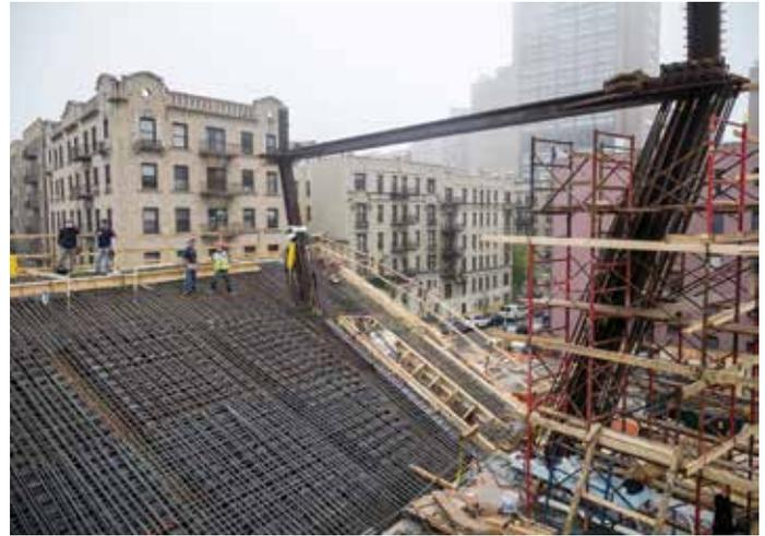
Figure 14. Combination of state-of-the-art materials and technology: void formers, high strength rebar, high strength concrete, and structural steel embedded in columns form the Auditorium structure at the base of the Cascade (Source: Matthew Melrose)
