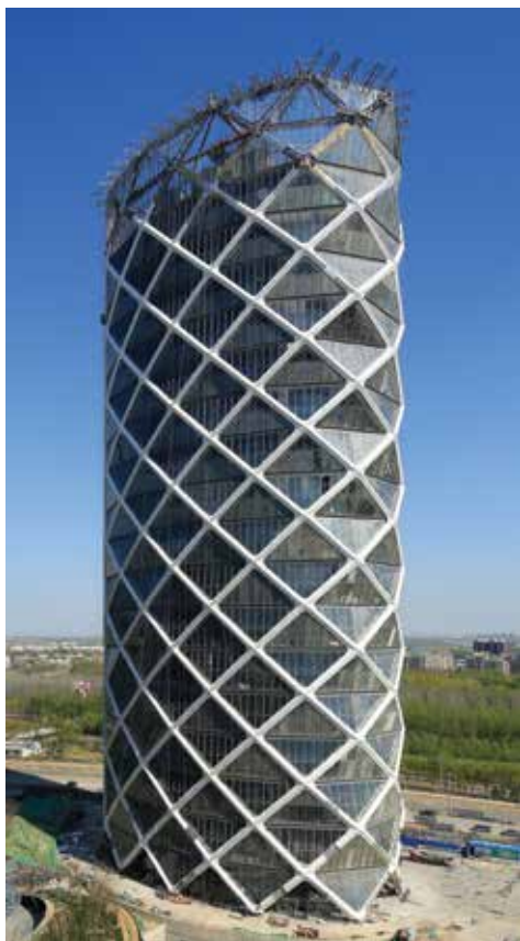
Figure 2. Poly International Plaza (Source: Skidmore, Owings & Merrill)
