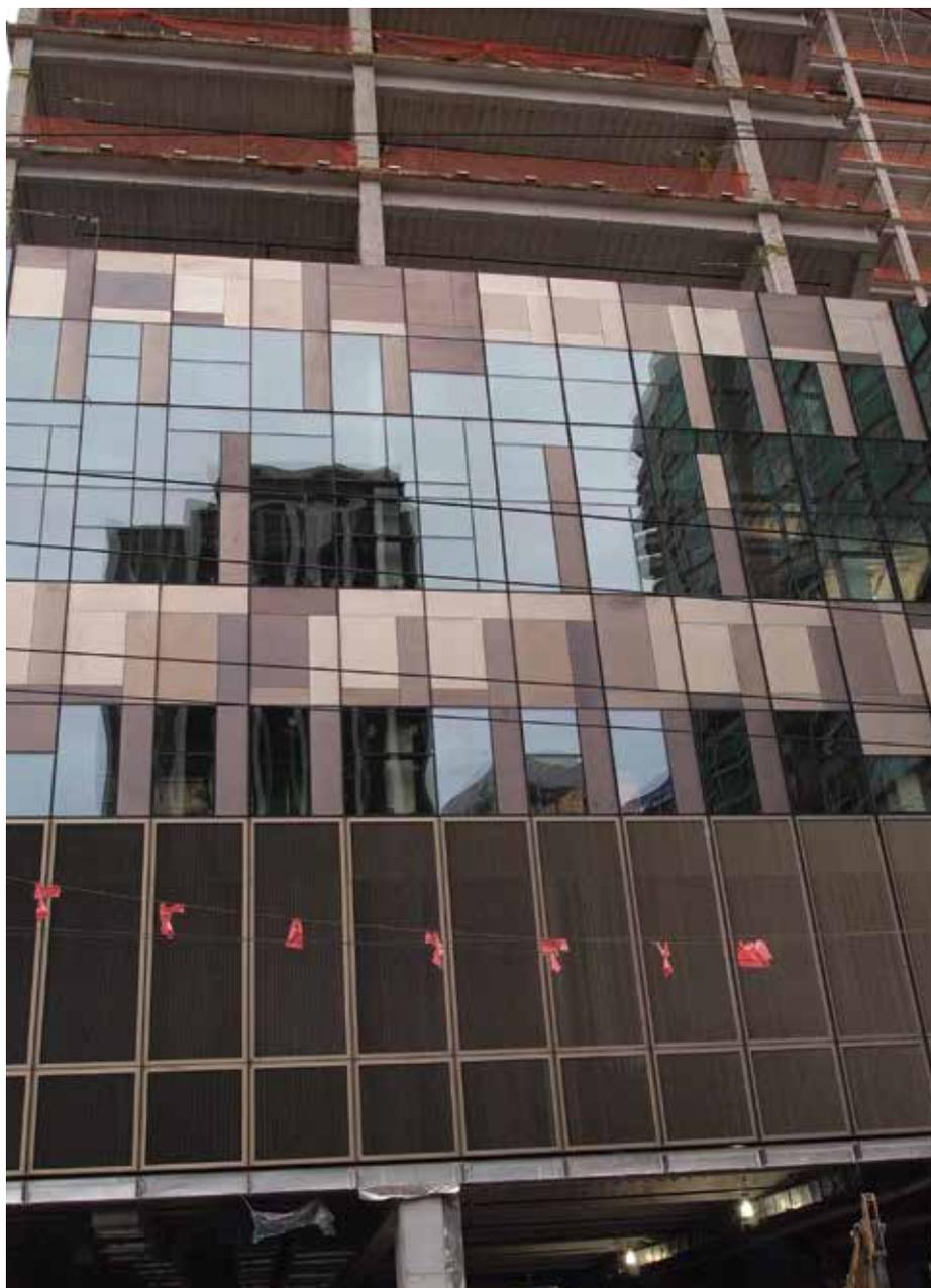
Figure 1. Installation of the electrochemically colored stainless steel panels on a corporate office building in Seattle, Washington, USA (Source: Walters & Wolf)
