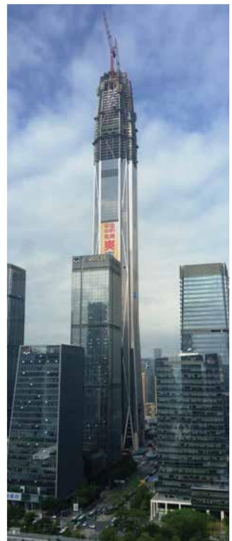
Figure 3. Almost completed curtain wall on Ping An International Finance Center (April 2015) (Source: Outokumpu)
