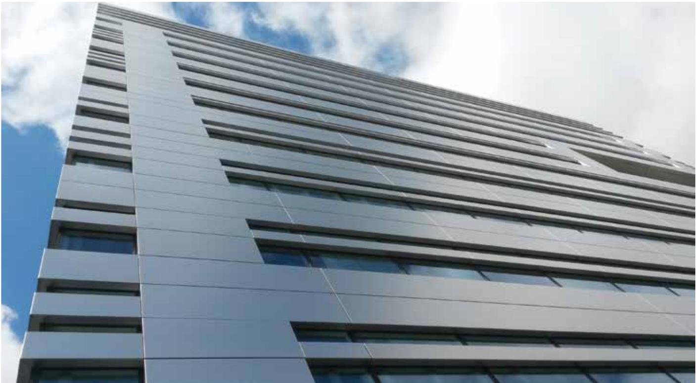
Figure 2. Stainless steel curtain wall on 5 Broadgate in London, UK (Source: Outokumpu)
