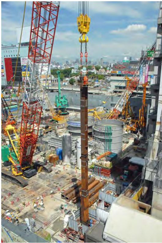
Figure 22. Underground piled column pre-erection method.
