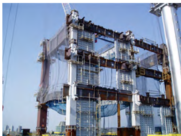
Figure 13. Erection of corrugated steel plate walls.
