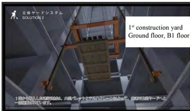
Figure 5. Large telfer crane at temporary opening.
