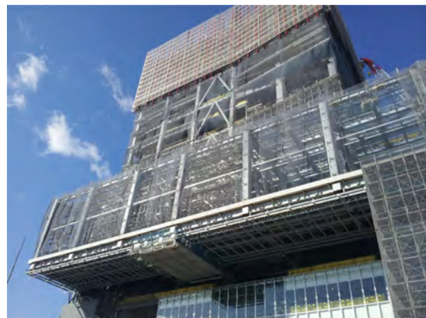
Figure 9. Suspended scaffolding for finishing.
