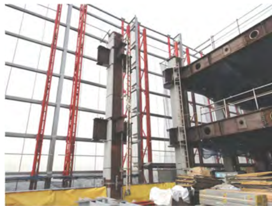
Figure 16. Steel erection within sliding cover.
