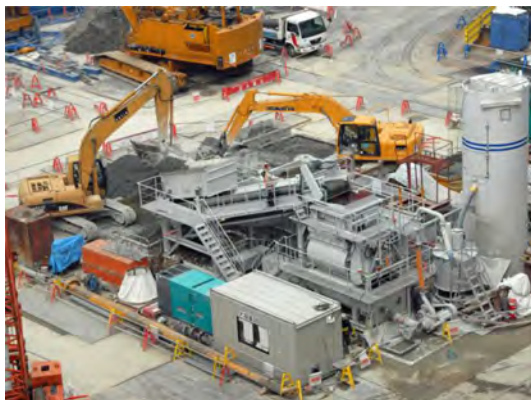
Figure 20. Soil cement plant at site.
