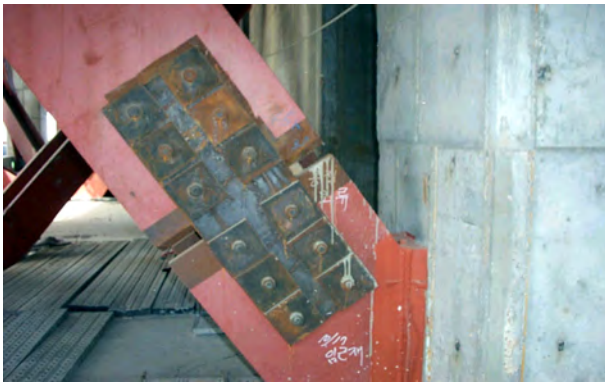
Figure 5. Delay joint (Hyperion I).
