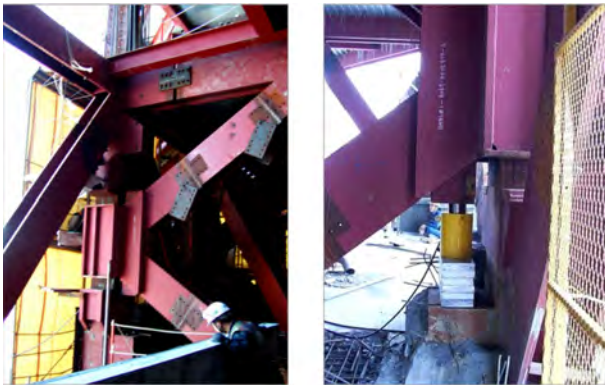
Figure 6. Adjustment joint (Hyperion I).
