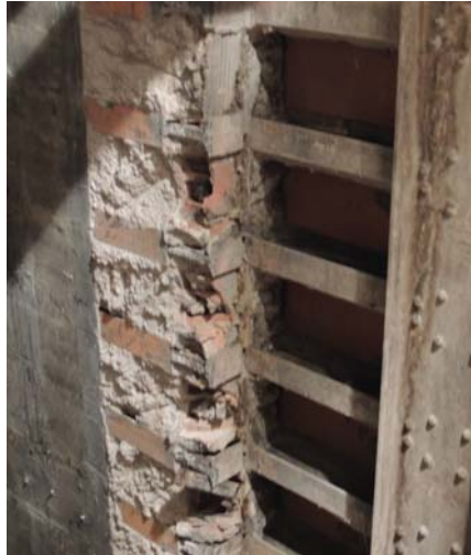
Figure 6. Existing shaft reinforcement.
