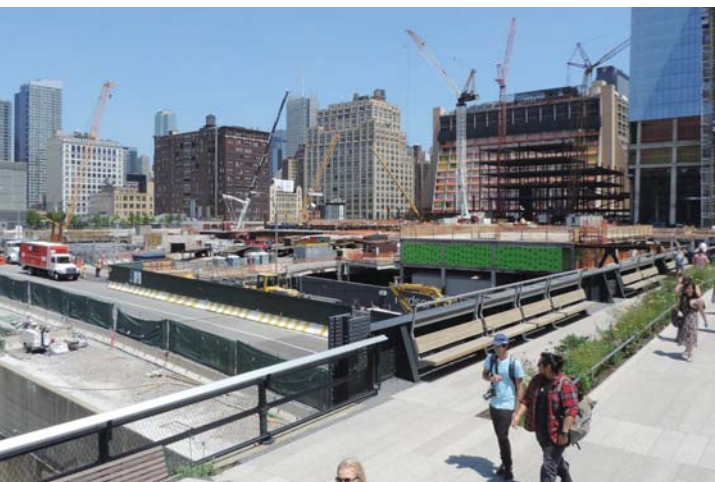
Figure 1. Hudson Yards – view from 30th Street High Line, July 2015. © Jim Henderson
