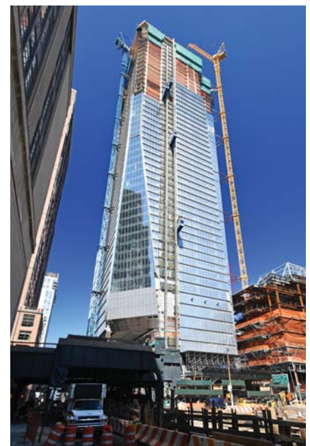
Figure 3. 10 Hudson Yards nearly tops out. Photo taken on September 18, 2015. © Royce Douglas
