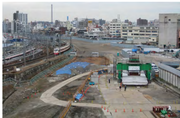
Figure 2.10. Pull-out test of a wall pile.
