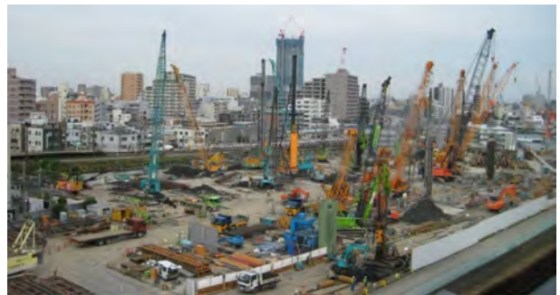
Figure 3.4. Construction of continuous underground wall pile.
