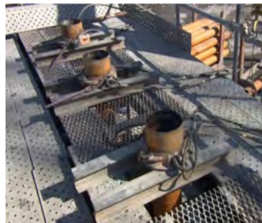
Figure 3.19. Setting tremie pipes.
