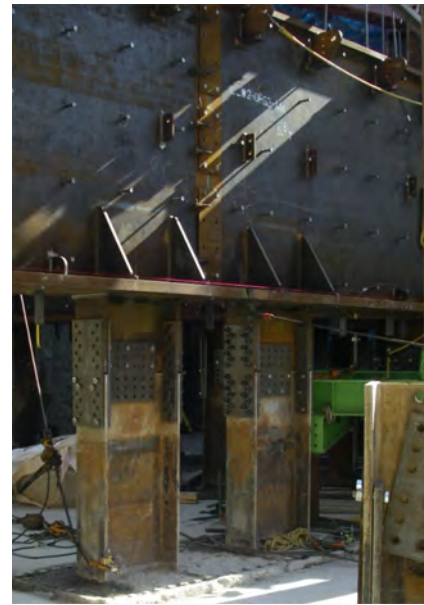
Figure 3.23. Foundation steel girder.
