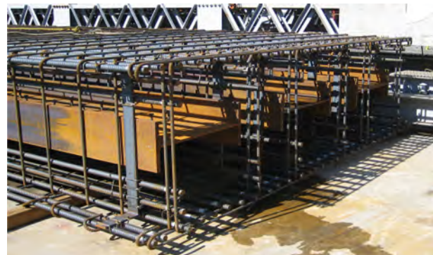
Figure 3.13. Cage of steel frame and bar.
