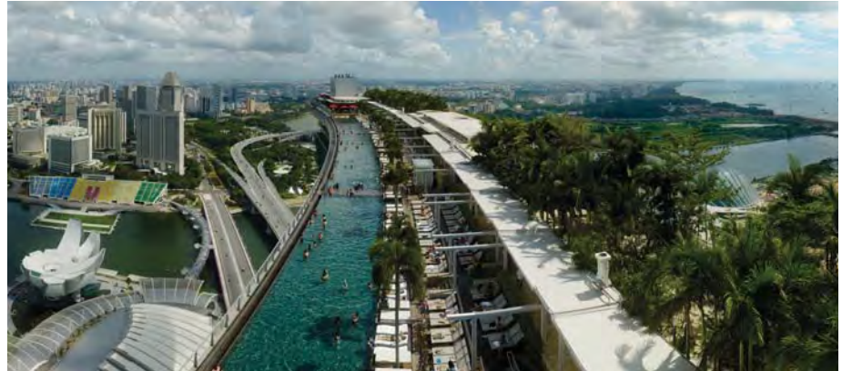
Figure 4. Marina Bay Sands, Singapore, takes full advantage of its connecting sky deck, including a spectacular infinity pool. © Timothy Hursley
