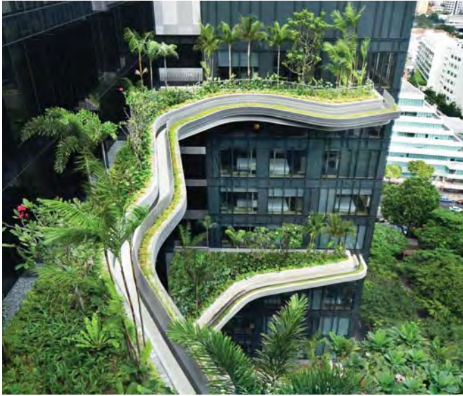
Figure 8. PARKROYAL on Pickering, Singapore dramatically brings the lush greenery of its surroundings into the sky with terraces, water features, and overhangs. © PatrickBingham-Hall
