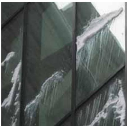
Figure 1. Example of snow and ice freezing on vision glass panel. © NMI
