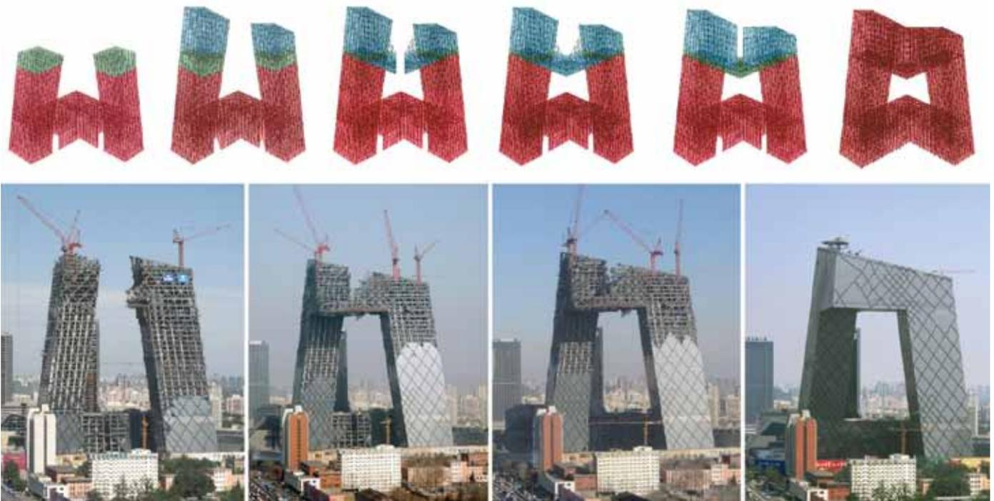
Figure 9: CCTV construction sequence. © Arup
