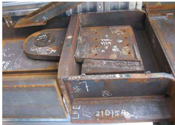
Figure 17. Middle outrigger girder pin at column.
