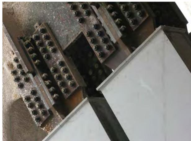
**Figure 8.** Quadruple BRBs bolted to gussets at upper connections. Note access to inner bolts.
