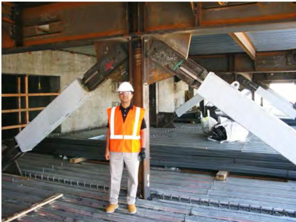
**Figure 9.** Single BRBs at middle outrigger use field welded splice plate connections. The red X shows a delayed connection.
