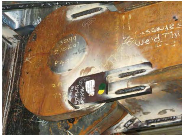
Figure 16. Middle outrigger girder pin at core wall.
