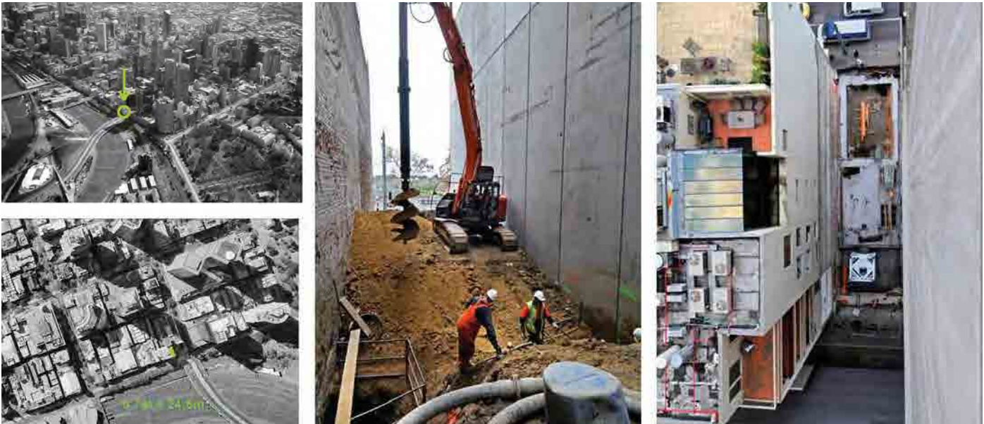
Figure 4. Early construction works on the site. © Fender Katsalidis Architects
