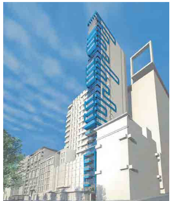
Figure 3. Phoenix Apartments final scheme showing slenderness ratio of 1 to 16. © Fender Katsalidis Architects
