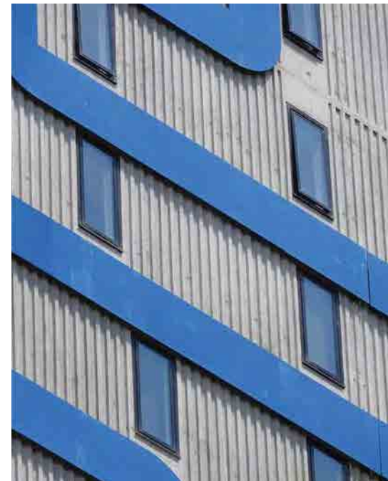
Figure 7. Close-up view of jump-form ribbed, in situ concrete façade.
