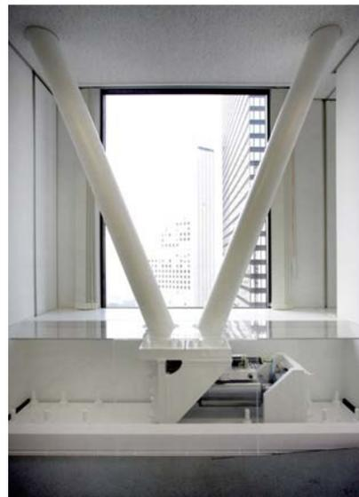
**Figure 9.** Picture of the oil damper.
