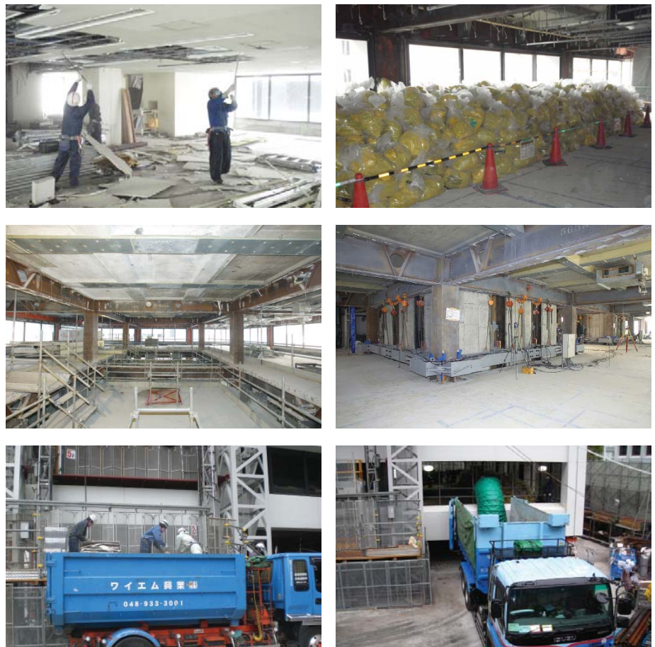
Figure 11. Interior and building demolition © Kajima
