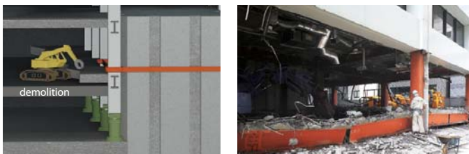
Figure 4. Demolition process © Kajima
