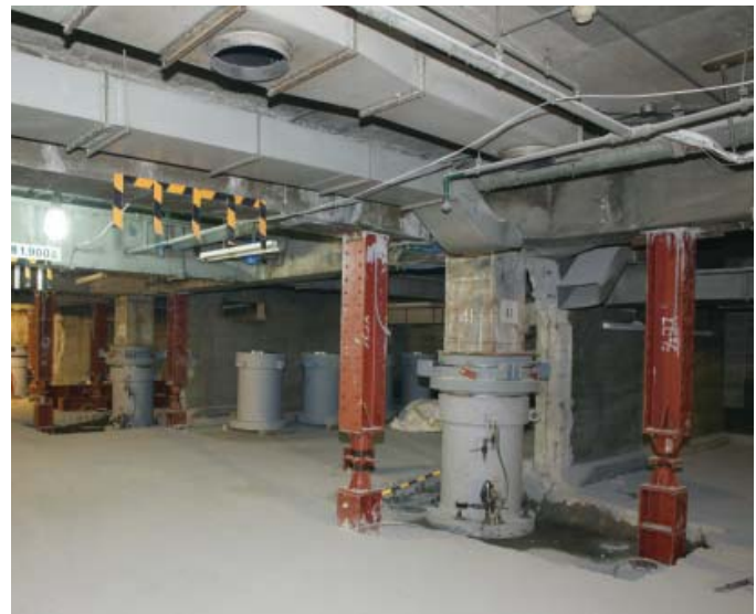
Figure 6. Temporary support columns © Kajima
