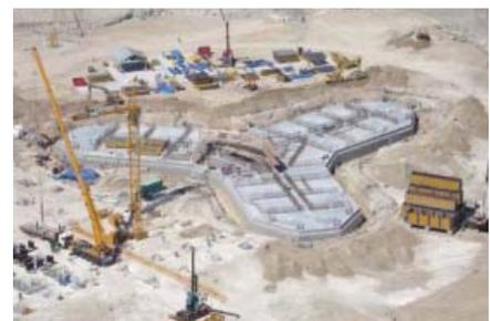
Figure 5. Raft construction © Samsung C&T
