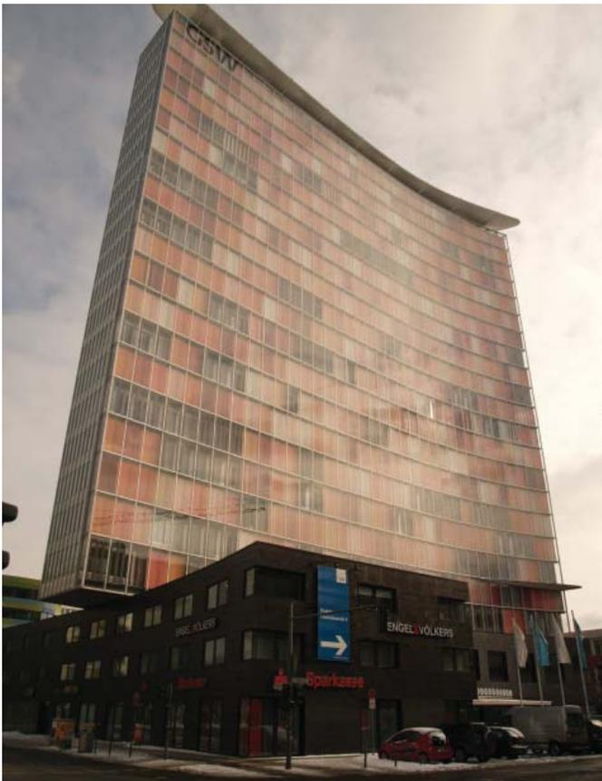
Figure 4. GSW Headquarters, Berlin – the building form of the narrow slab tall building, with movable shading devices on the west elevation within the operable double-skin façade, as part of the strategy for the natural ventilation © Carsten Ernest.
