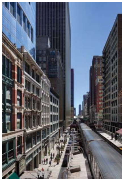
Figure 5. The restored façades integrated into the base of the Legacy tower, looking south along Wabash Avenue © Tom Rossiter Photography
