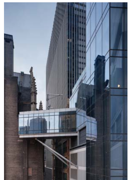
Figure 6. The cantilevered sky-bridge connecting the 13 th floor of the Legacy tower to the adjacent University Club © Tom Rossiter Photography
