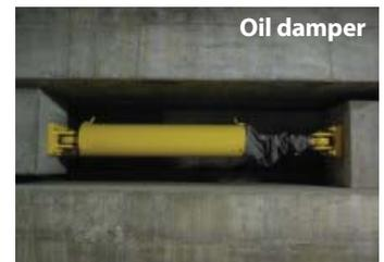
any slanting or stroke to the vibration control dampers when positioning the sky gardens, all planting and finishing of the gardens was first completed and then the vibration control dampers were fixed to the buildings.
