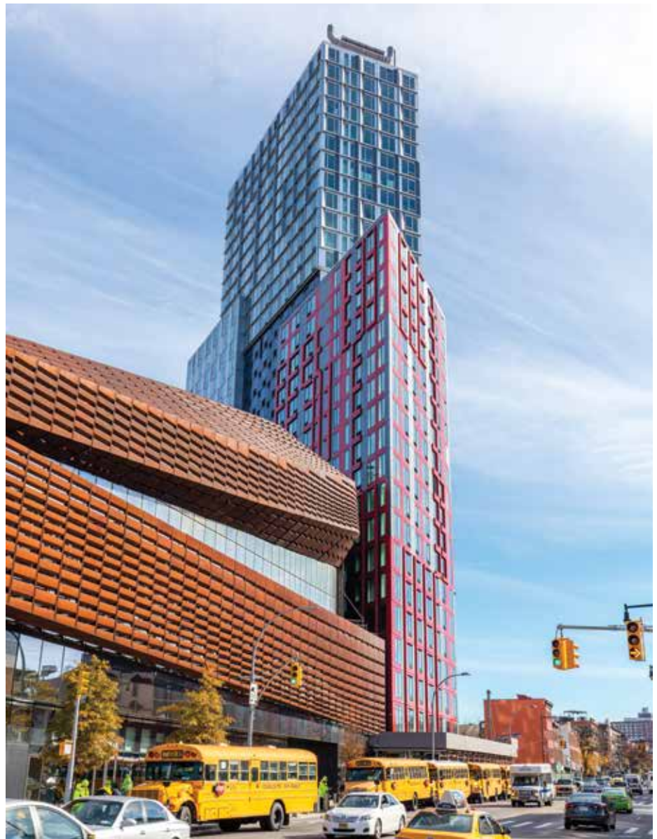
Figure 1. 461 Dean Street, New York. © SHoP Architects
