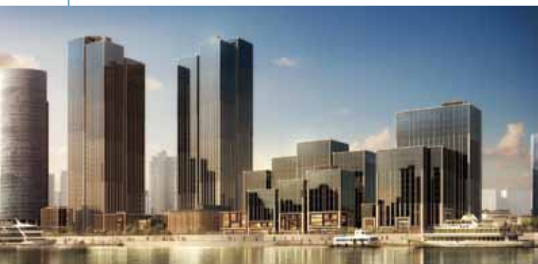
Bund Finance Center, Shanghai. © Bund Finance Center
