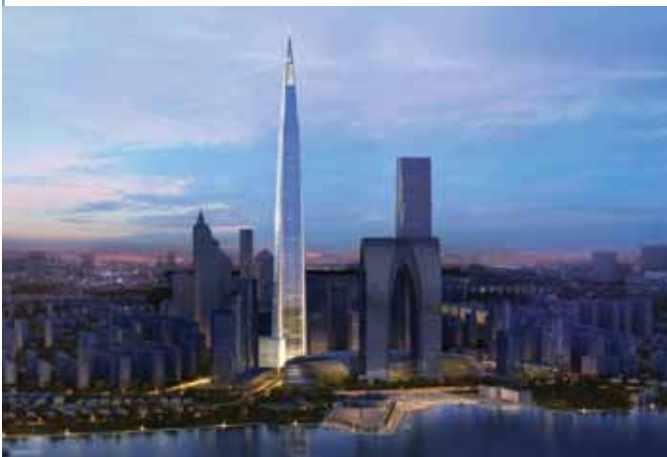
Suzhou Zhongnan Tower, Suzhou. © Zhongnan Group
