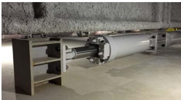
Photo 2. Damper with a locking mechanism.
