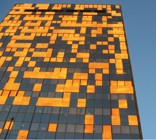
Figure 1. Brickell Avenue, Miami (2006) – plywood repair after Hurricane Wilma damaged the Colonial Bank building. © Jordan Fischer (cc by-sa)
