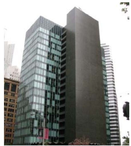
Figure 10. External service core of One Bush Street in San Francisco
