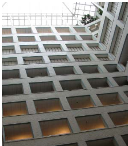
Figure 4. Light well of the Railway Exchange Building in Chicago. The internal walls were clad in white tiles in order to reflect the light into the offices located in the lower floors
