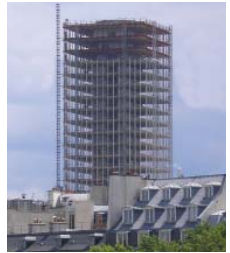
Figure 9. Restoration of the Université Paris 4 Building, Paris
