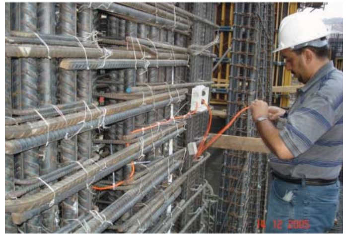
Figure 18. Installation of vibrating wire strain gauges
