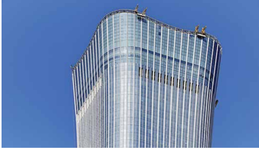
Figure 2. The facade of China Zun will be kept clean by two sets of building maintenance units - one at the top, shown here, and one at the "waist" or mid-section of the building. © Shuhe Photo
