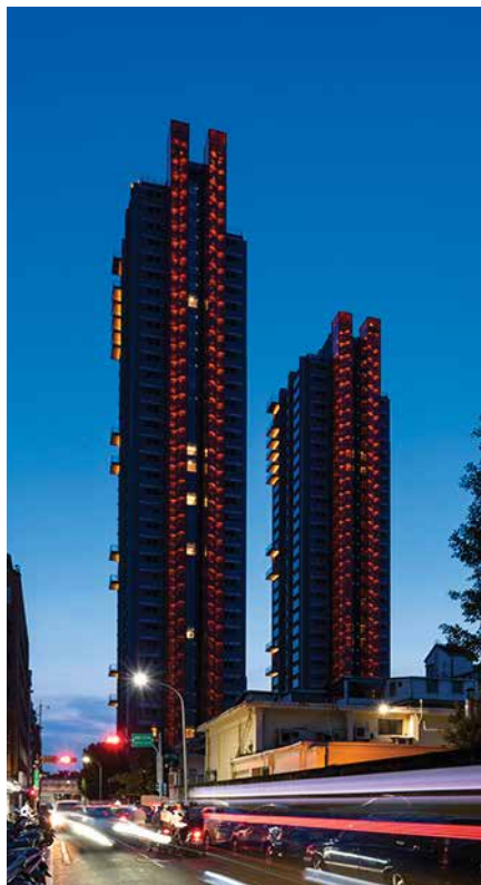
Figure 2. One Park Taipei, Taipei. © Rogers Stirk Harbour + Partners
