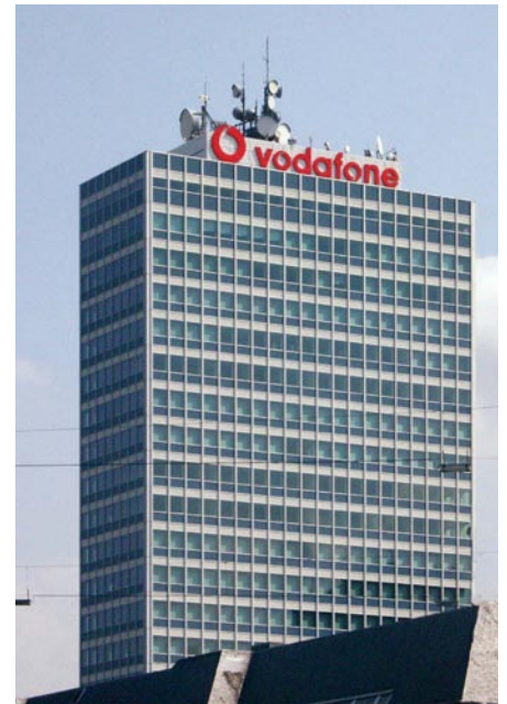
Figure 4. Mannesmann-Hochhaus, Düsseldorf, Paul Schneider-Esleben, 1954-57. © Raimond Spekking
