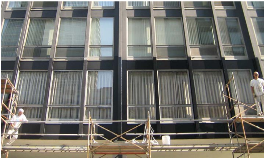
Figure 7. Façade painting mock-up. © Harboe Architects
