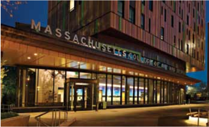
Figure 3. Main entrance. © Chuck Choi
