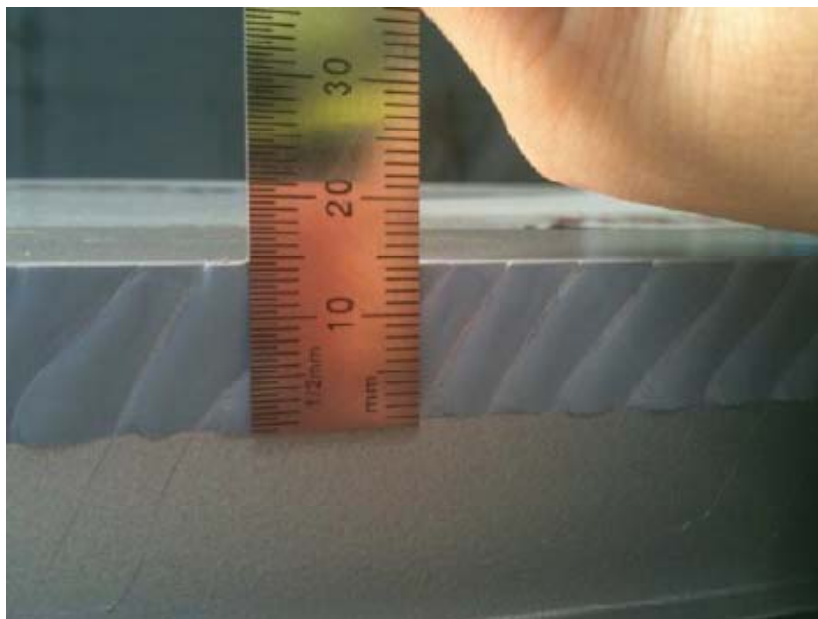
Picture 2. Measuring required structural bite dimension upon deglazing for curtainwall units
