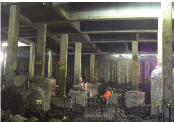
Figure 4. Top down construction at The Shard. © WSP
