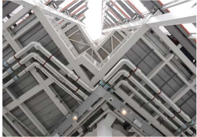
Figure 7. Steel framed structure above the residential levels. © Terri Meyer Boake
