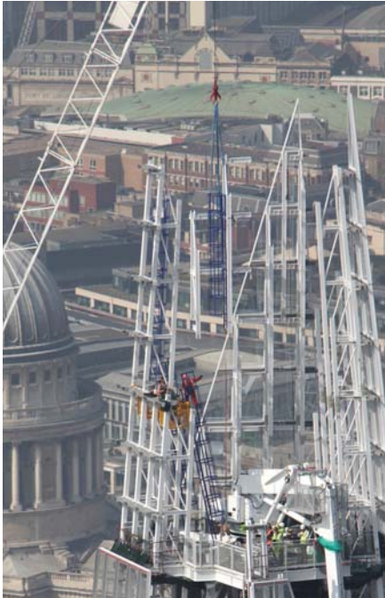
Figure 8. Installing the steel spire. © Mace
