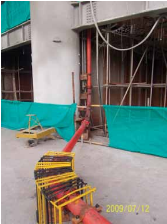
Figure 8. Connection example of concrete pump pipe and steel column (source: Yang Yaohui Gao Junfeng & Wang Jing) 图8. 混凝土泵管与钢柱连接实例图 (出自: 杨耀辉)
