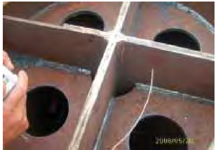
Figure 7. Grouting hole (source: Yang Yaohui Gao Junfeng & Wang Jing) 图7. 灌浆孔 (出自: 杨耀辉)
