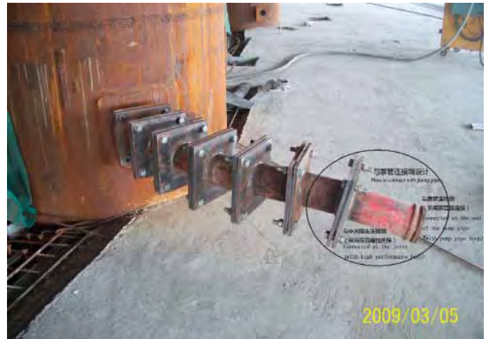
Figure 4. Lifting interface with pump pipe connecting section (source: Yang Yaohui Gao Junfeng & Wang Jing) 图4. 与泵管连接端顶升接口 (出自: 杨耀辉)
