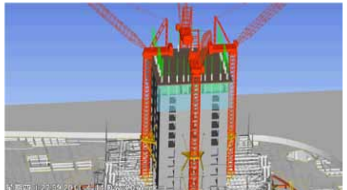
Figure 6. Simulation of the construction site in 4D (Source: Shanghai Tower Construction and Development Co., Ltd.) 图6. 施工4D模拟 (出自: 上海中心大厦建设发展有限公司)
