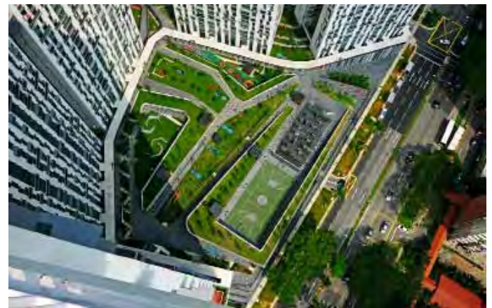
Figure 3. Raised new ground: stitching seamlessly to the city ground plane while providing a distinct threshold for a transition from the public to private realm. (Source: ARC Studio Architecture + Urbanism) 图3. 抬高的新地面层: 与城市地面完美衔接同时在公共空间和私人空间之间有明显的过度。(出自: ARC Studio Architecture + Urbanism)
