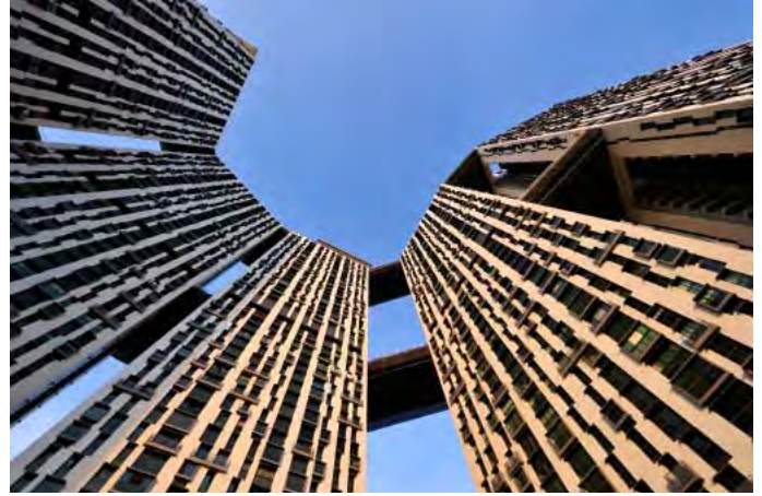
Figure 7. Pre-fabricated facade: the pattern structure reduces the perceived mass of the building. (Source: ARC Studio Architecture + Urbanism)
