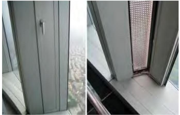
Figure 6. The details of operable walls in Zifeng Tower (Source: Jianqiang Li)
