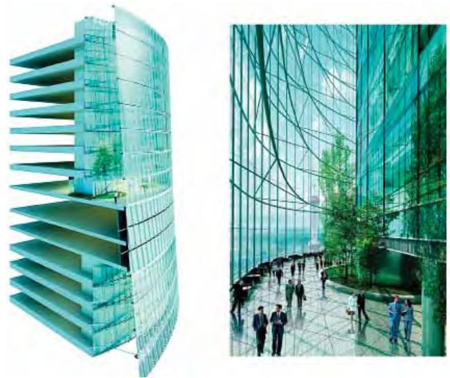
Figure 8. The buffer space in Shanghai tower (Source: <http://openingbuilding.com>)
