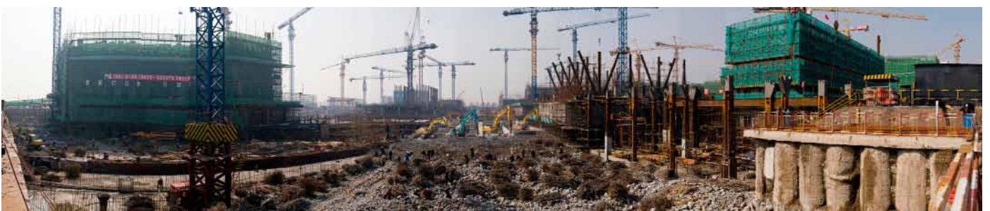
Figure 10: Construction Well Underway, 2012 (Source: SOM)
