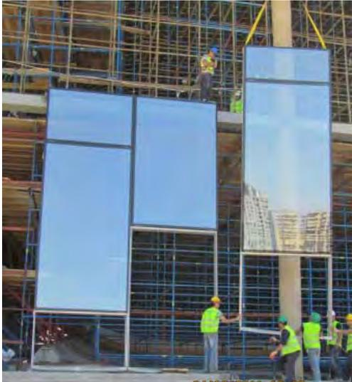
Figure 9. Heydar Aliyev Center – structural bonding unitized 7.5 x 2.5m façade panels
