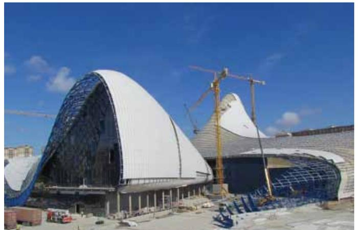
Figure 10. Heydar Aliyev Center – Construction of the 3D envelope in functional layers
