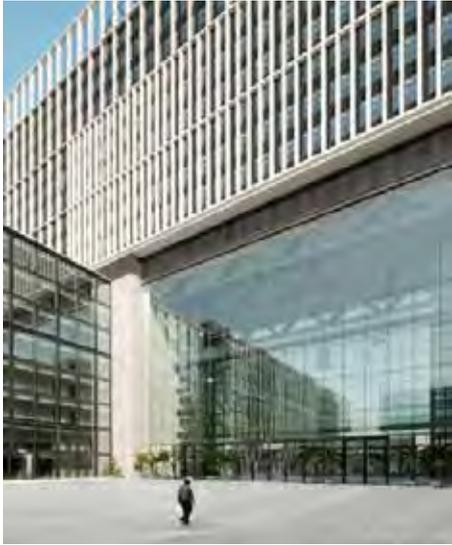
Figure 4. Office High Rise Hanoi – partial view of main building with cable-façade lobby
