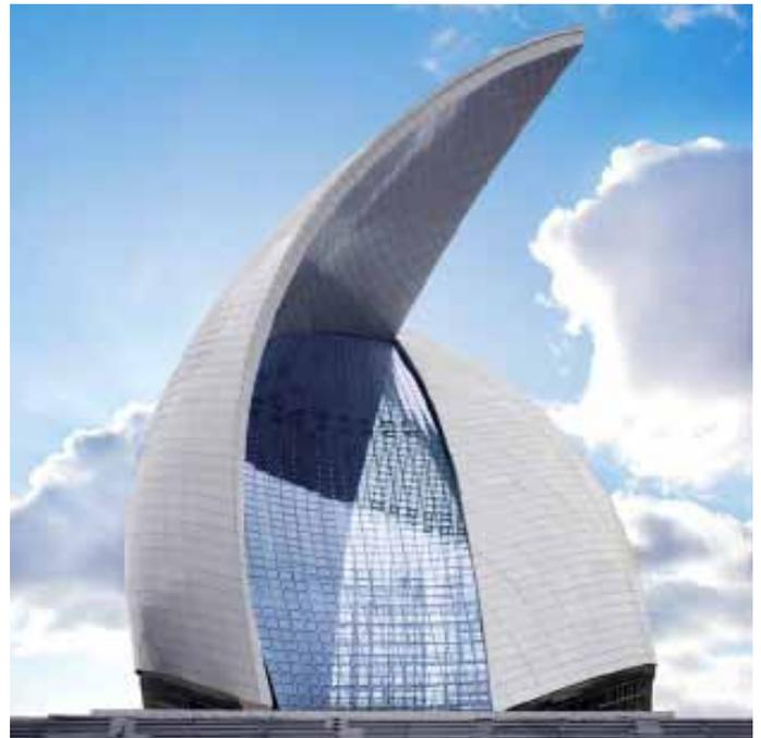
Figure 6. Maritime Museum Lingang – view showing the two structural “sails” and the cable-net in between
