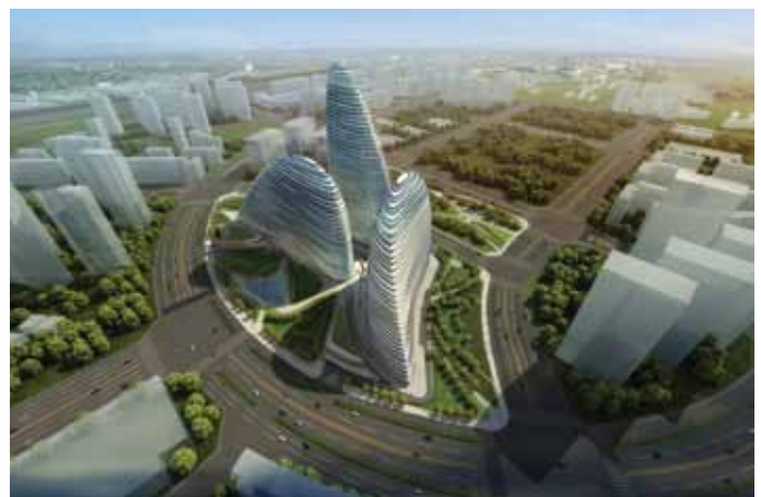
Figure 5. Overall aerial view of the Wangjing SOHO project. 图5. 望京SOHO空中纵览图
