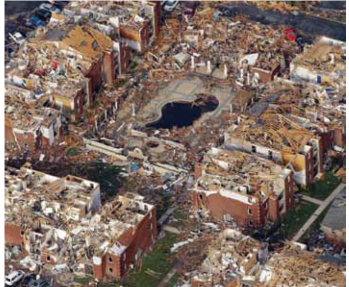
Figure 7. Brick Cladding with Wood-Framed Walls and Roofs (source: Charlie Riedel, Associate Press)
