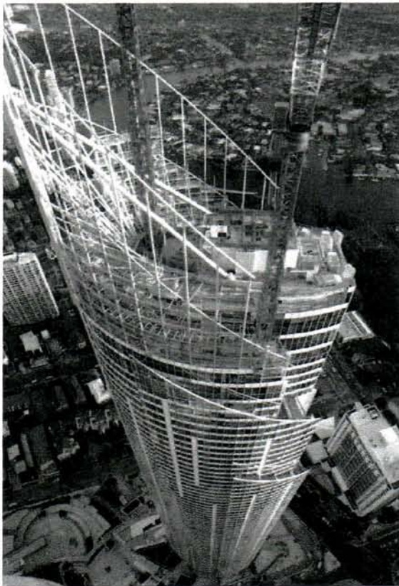
Figure 21: Residential buildings in the 300-m range generate new serviceability and partition design concerns. Sunland Designs' Q1 in Surfers Paradise, Australia, was wind-tunnel tested by an Australian wind-engineering firm.
