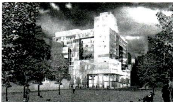
Figure 19: The Genzyme Headquarters in Boston, Massachusetts, was analyzed for cladding pressures when selected critical windows were assumed open during a design storm.
