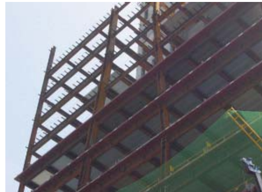
Fig. 11. Construction of Sloping Column in the West Side 7th~11th Floors
