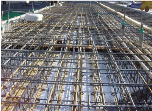
Fig. 8. Pre-Assembled Steel Deck System
