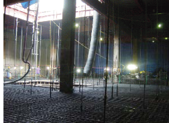
Fig. 6. Construction in Sub-ground Levels with NSTD Method hanged with \phi 25\text{mm}
