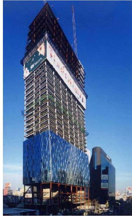
Fig. 21. Curtain Wall Construction in NOV., 2003
