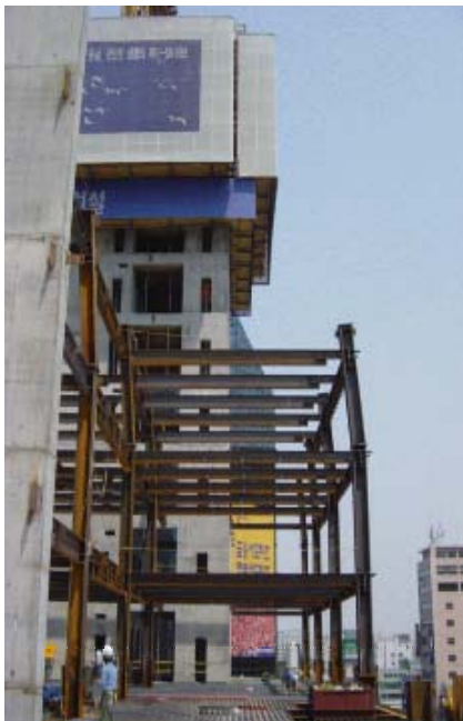
Fig. 9. Construction of Sloping Column in the Front Side 7th Floor
