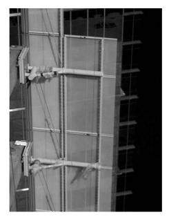
Figure 25 Façade fin cantilevered steel framing.
