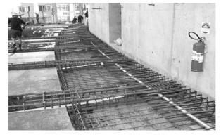
Figure 17 Typical floor band connection to the outer core wall.
