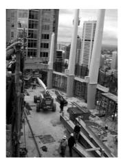
Figure 29 West sail needle erection.
