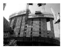
Figure 7 Core jumpform construction.
