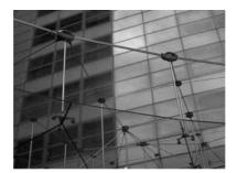
Figure 32 Piazza canopy spider and hanger connections.
