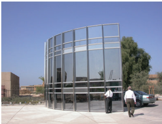
Figure 18. Tower exterior wall visual mock-up
