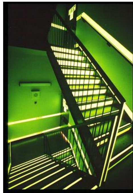
Figure 6. – Photoluminescent stair/path lighting (source: irc.nrc-cnrc.gc.ca)
